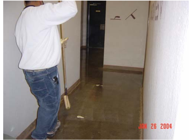
Applying first coat of epoxy, having a uniform film is important.
