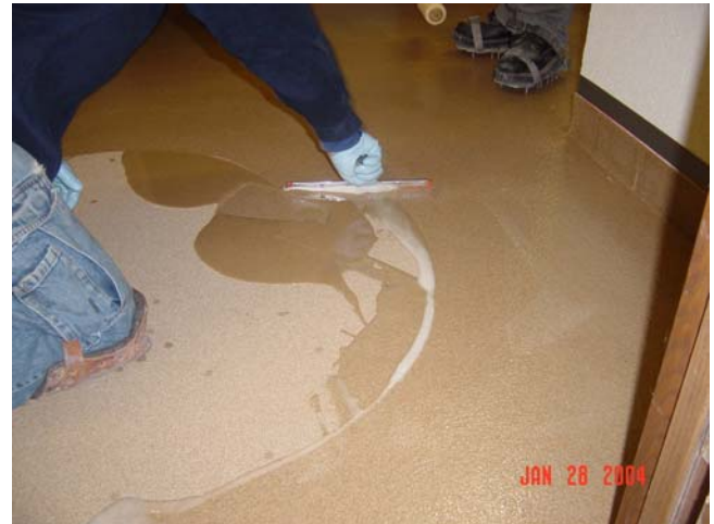
Applying first coat of epoxy, having a uniform film is important.
