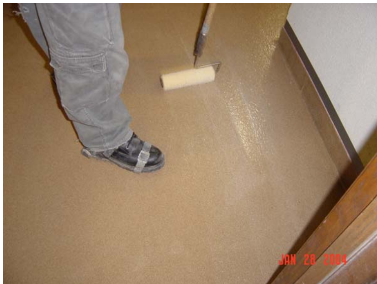
Applying aggregate
