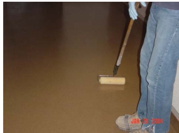
Applying Third and Top Coat of Epoxy and Back Rolling.
