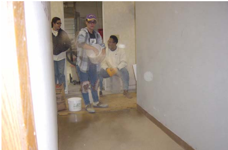
Applying Second coat of aggregate.
