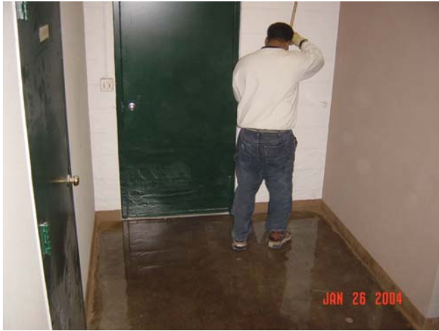
Applying first coat of epoxy, having a uniform film is important.
