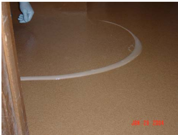
Applying Third and Top Coat of Epoxy and Back Rolling.
